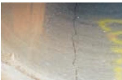
cracks, leaking joints and D ring cracking. Who bears the cost of such a dig up?
