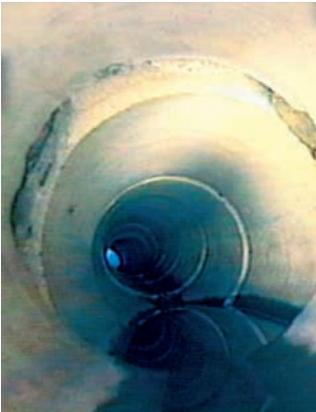
**Misaligned pipe - offset joints**
