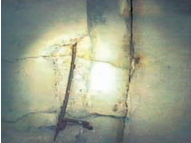
**Exposed rebar and cracked bell**
