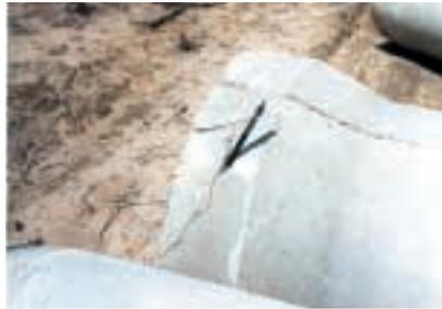
**Severe damage and exposed reinforcing steel**
