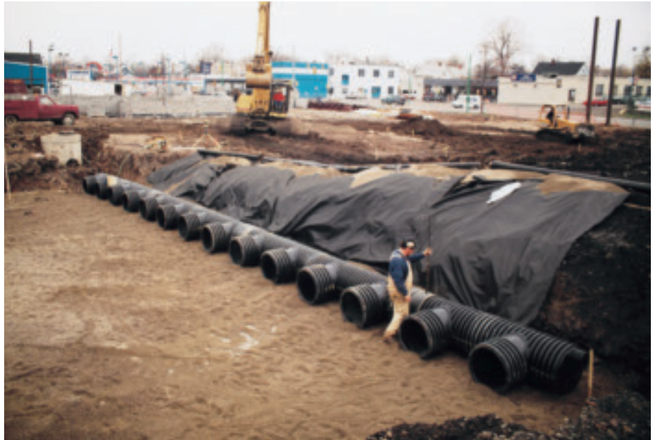
Underground retention/detention systems use ADS large diameter pipe and Propex geotextiles to effectively control stormwater runoff.
