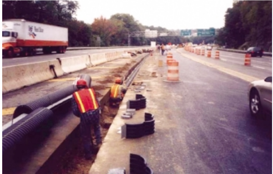
Heavy equipment is not required to set DURASLOT drains in place. Long, lightweight sections and easy-to-use coupler bands cut installation time significantly.
