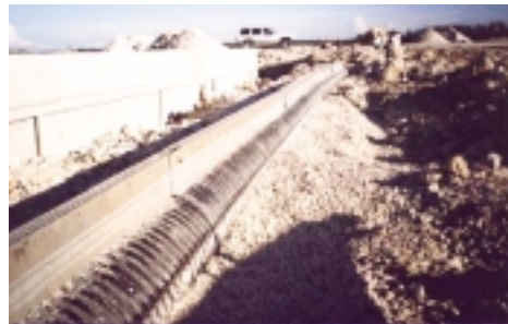
Heavy equipment is not required to set DURASLOT drains in place. Long, lightweight sections and easy-to-use coupler bands cut installation time significantly.
